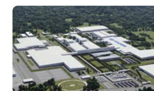
Plant #3 — Pune, Maharashtra
