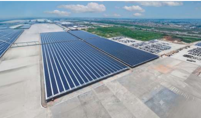
A view of the in-house solar power generation facility
