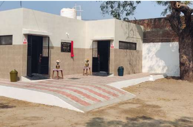
Toilet Block Constructed at Local Community School
