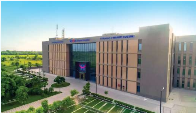
Multi-Specialty hospital at Sitapur, Gujarat
