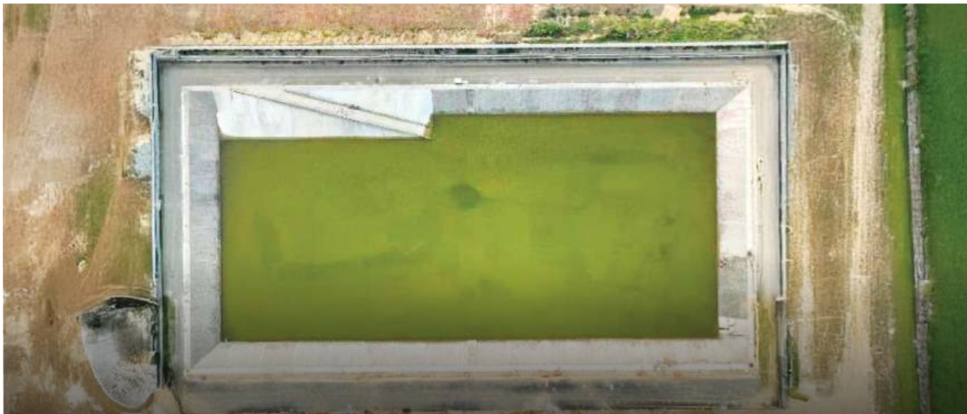
Rainwater storage facility at Kharkhoda manufacturing plant
