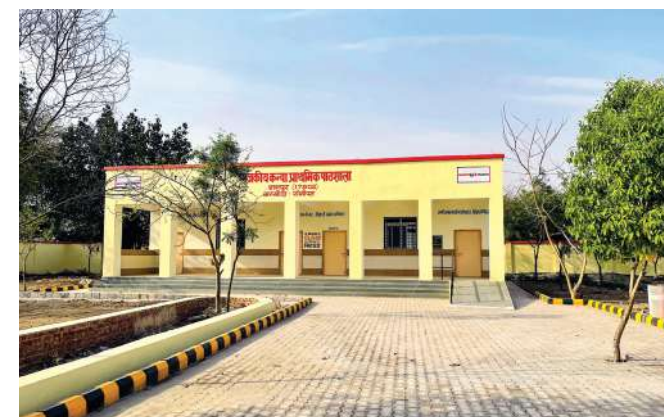
Classrooms constructed at one of the government schools supported
