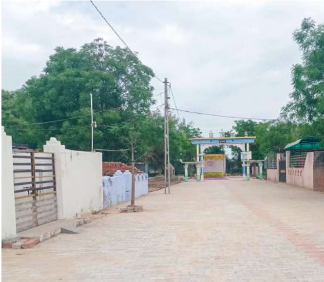
Paved road constructed at one of the project villages
