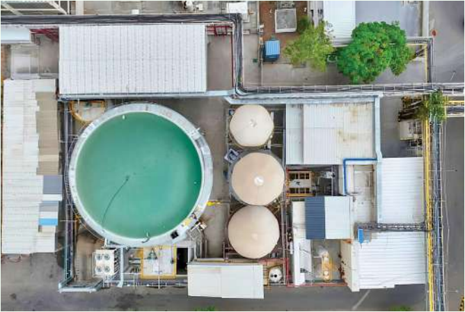
Biogas plant at Manesar facility
