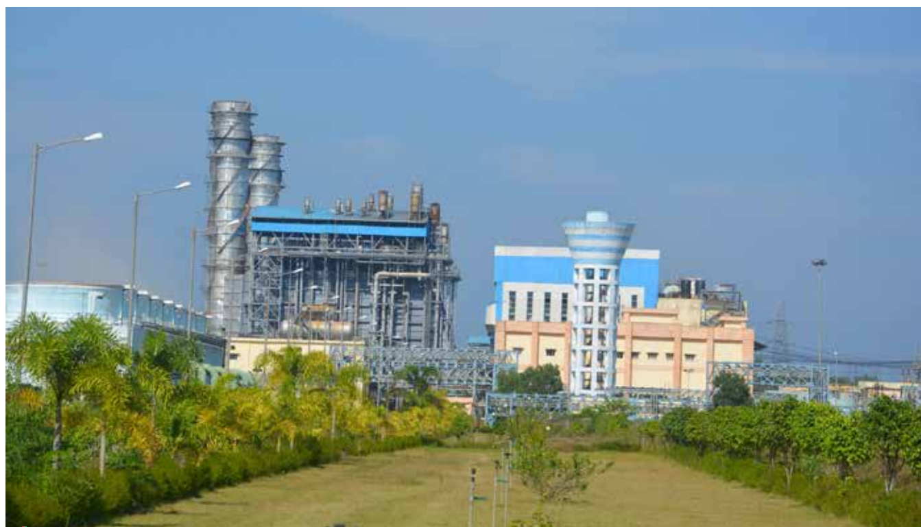
Powering the Northeast, illuminating homes and inspiring hope: ONGC Tripura Power Company
