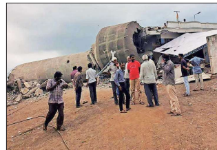
A grab from a video purportedly showing the collapsed tank. No person was injured in the mishap, the village sarpanch said.
