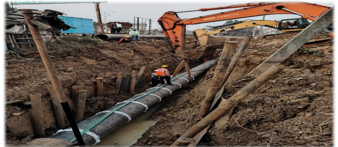
Setting up slurry pipeline
