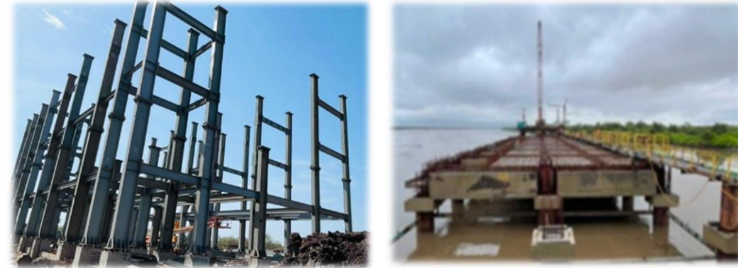
Expansion work at Dharamtar Port
