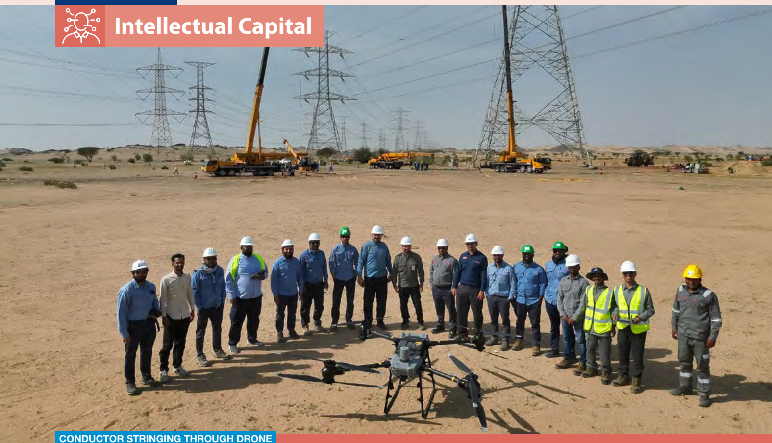
CONDUCTOR STRINGING THROUGH DRONE
