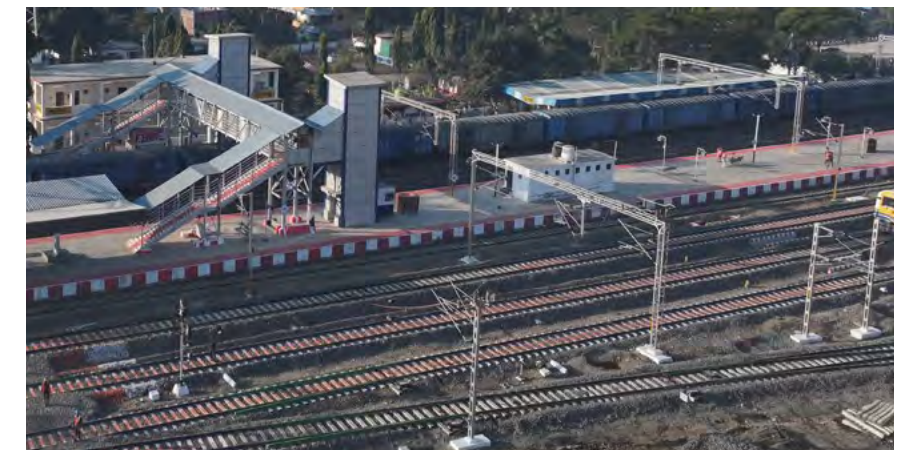
DOUBLING LINE AT NAGPUR-ITARSI RAILWAY SECTION, MADHYA PRADESH, INDIA
