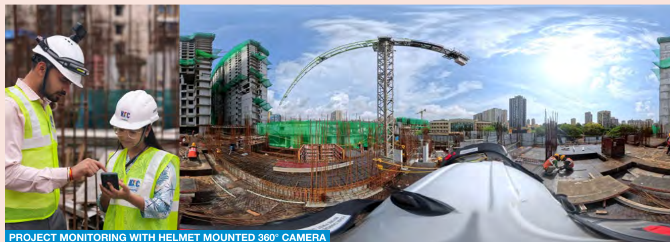
PROJECT MONITORING WITH HELMET MOUNTED 360° CAMERA
