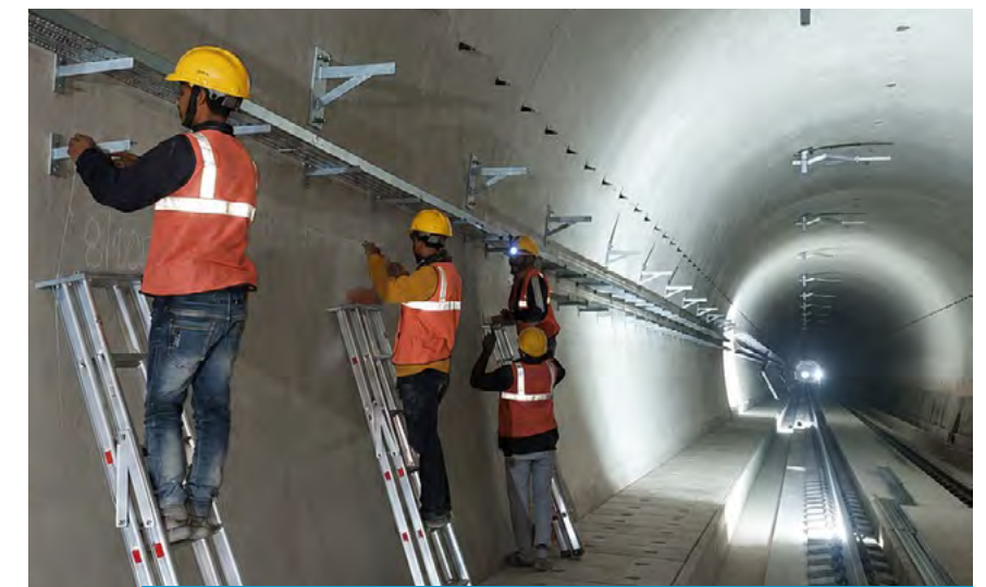
TUNNEL VENTILATION WORK, SIVOK-RANGPO TUNNEL, ASSAM, INDIA
