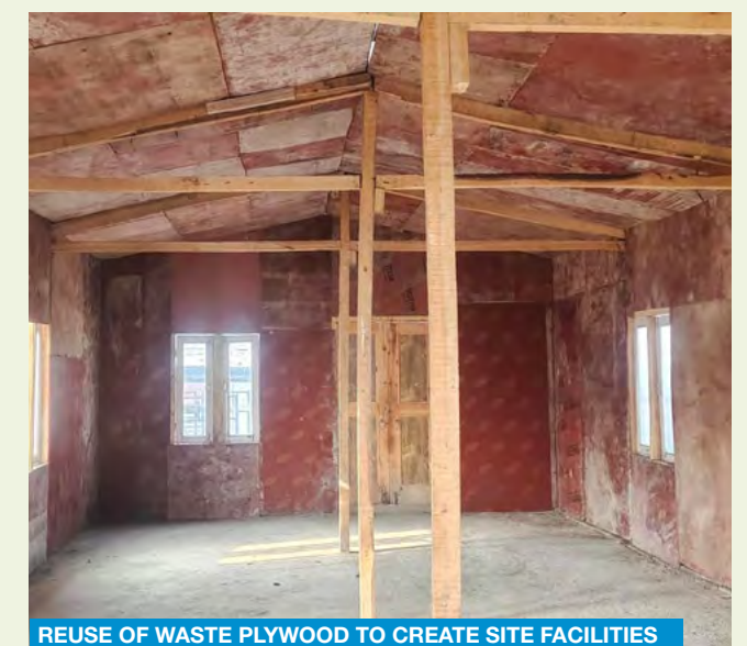
REUSE OF WASTE PLYWOOD TO CREATE SITE FACILITIES
