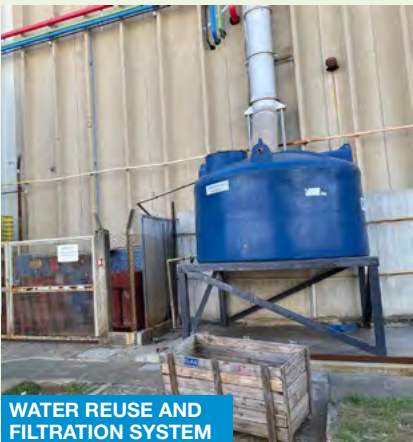
AC WATER HARVESTING SYSTEM AT A PROJECT SITE
