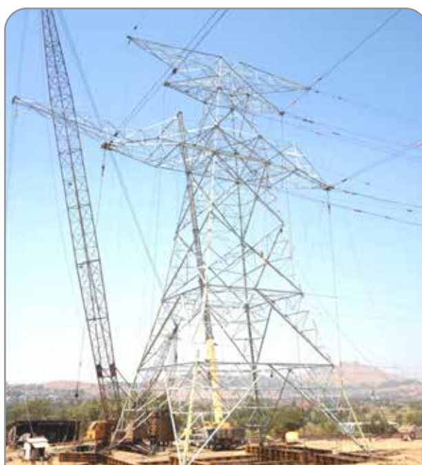
Power Grid Corporation of India Ltd. Project: 800kV HVDC Hexa ACSR Lapwing (Wind Zone – 4, RL-2) Date of testing: 12/03/2026 Weight of Tower:- 58.2 Mt Height : 48.5 Mtrs
