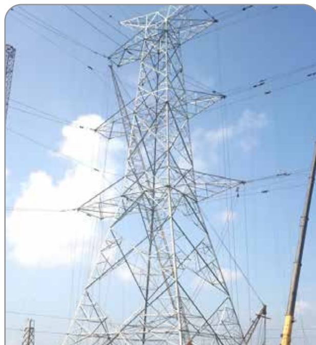
Resonia Limited Project: 765kV Anantapur -II REZ Transmission Limited Date of testing: 28/10/2025 Weight of Tower:- 70.79 Mt Height : 70.35 Mtrs
