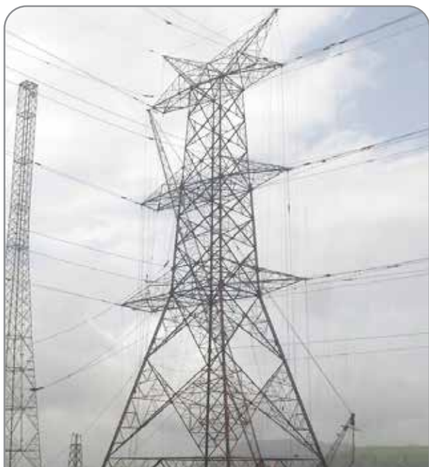
Reliance Industries Limited, Mumbai Project: 765kV Captive Power Transmission Line from Kutch – Z2 Parcel to JMD; Date of testing: 19/07/2025 Weight of Tower :- 105MT Height : 71 Mtrs
