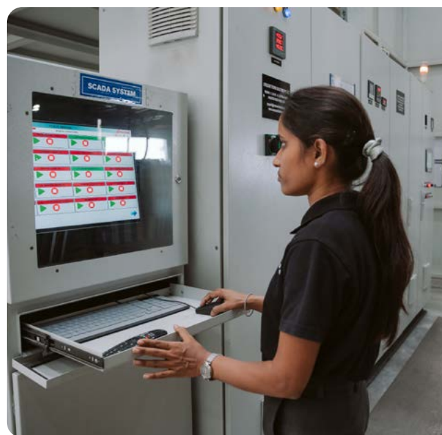
Operating SCADA system to monitor the powder coating processes, Chh. Sambhajnagar
