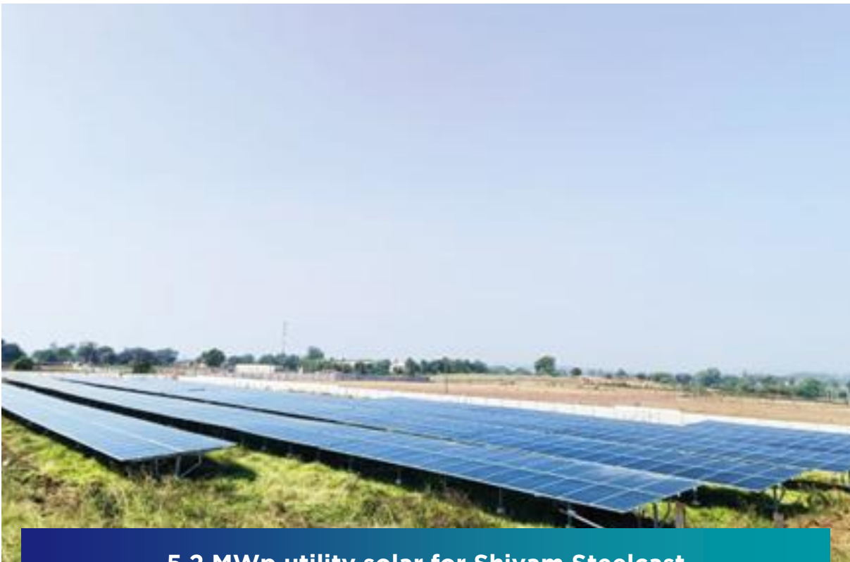
5.2 MWp utility solar for Shivam Steelcast
