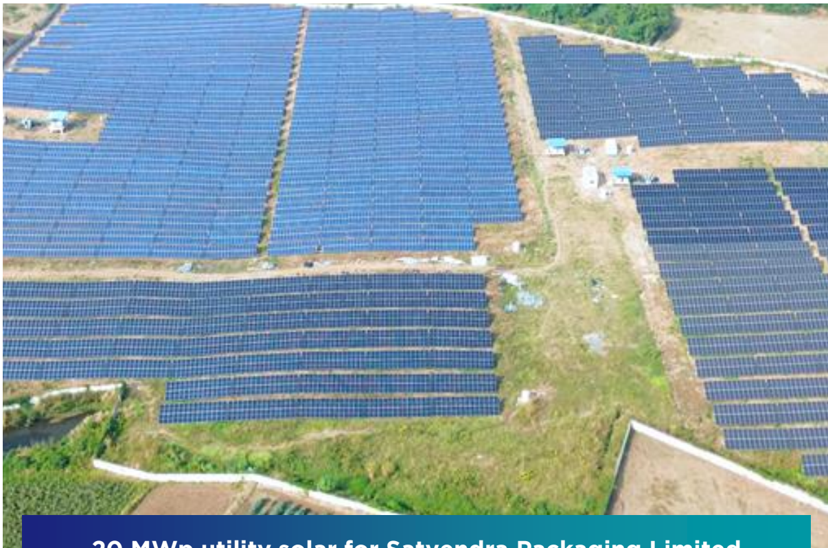
20 MWp utility solar for Satyendra Packaging Limited
