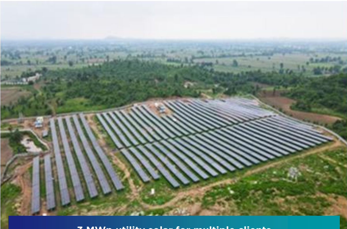
3 MWp utility solar for multiple clients
