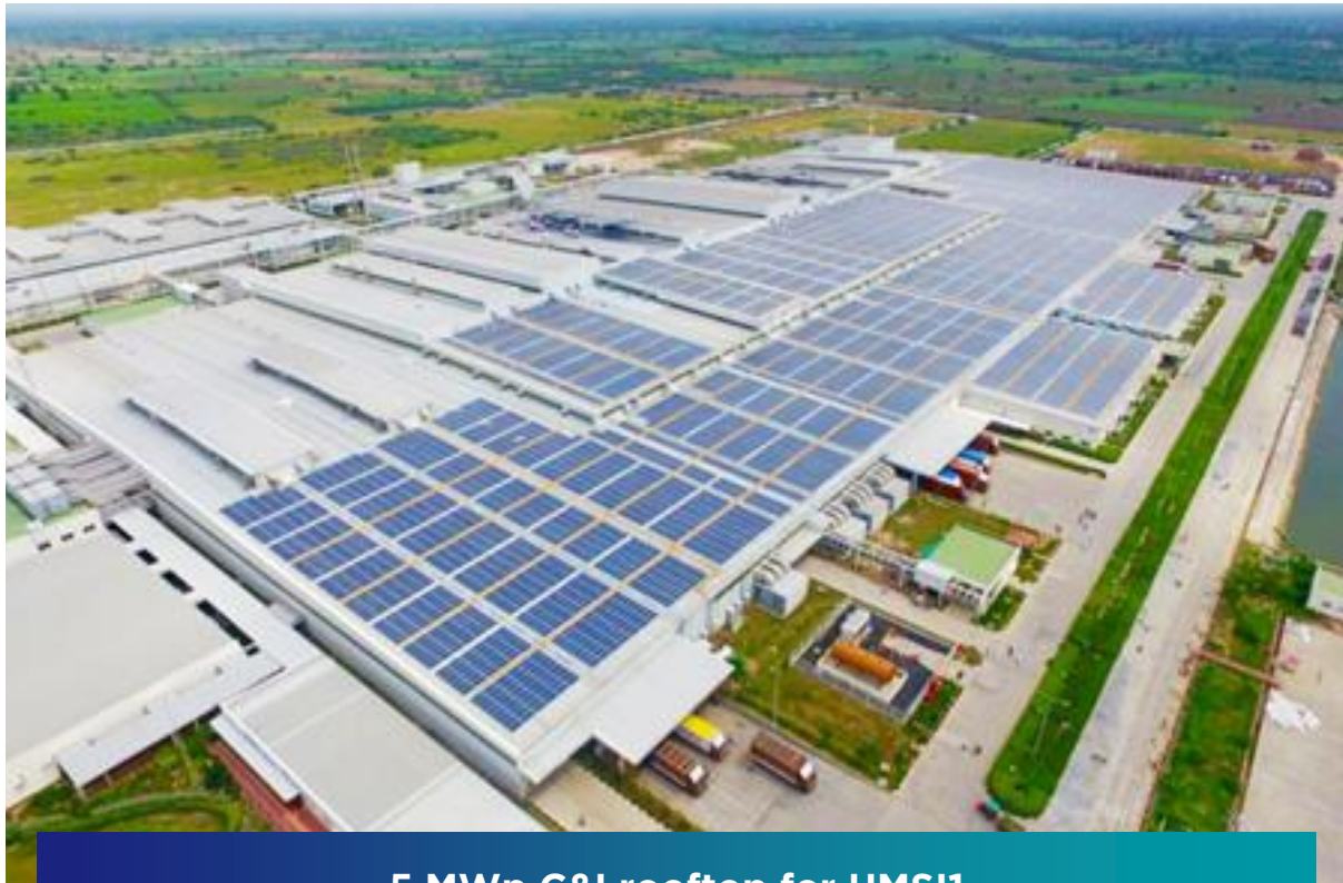
5 MWp C&I rooftop for HMSI1
