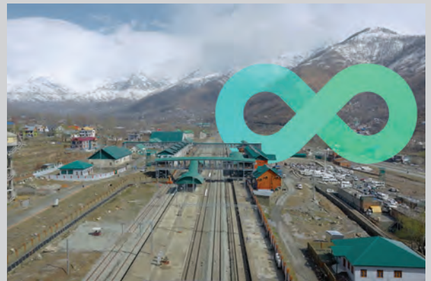
Siemens Limited completed India's first Rigid Overhead Catenary System on the challenging 42-km Kashmir railway route through Pir Panjal range in a record 16 months.
