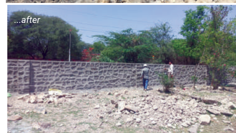
Repair of Boundary Wall
