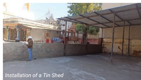
Installation of a Tin Shed Repair and strengthening of the Anganwadi Building, including renovation of the boundary wall
