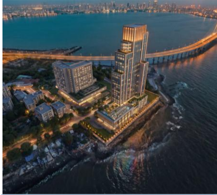
Taj Bandstand (95% Excavation completed)
